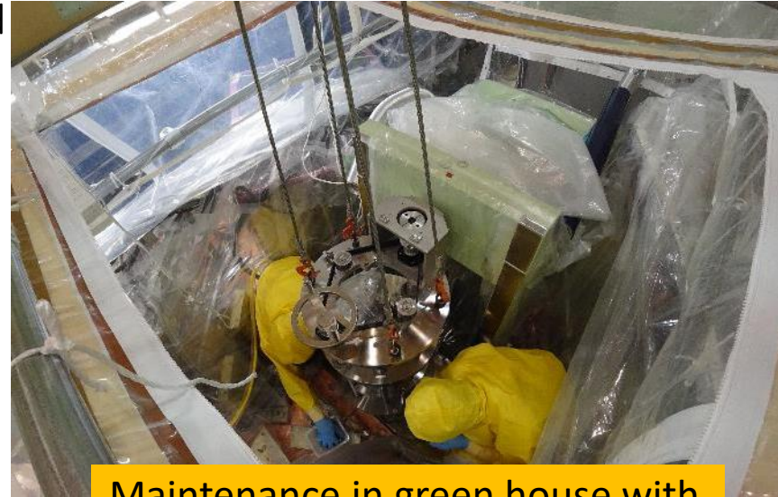
Maintenance in green house with anorack suits & airline mask.
