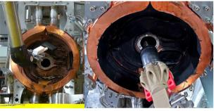
Figure 6: Target remote work: heat exchanger coating (left); bearing cartridge replacement (right).
